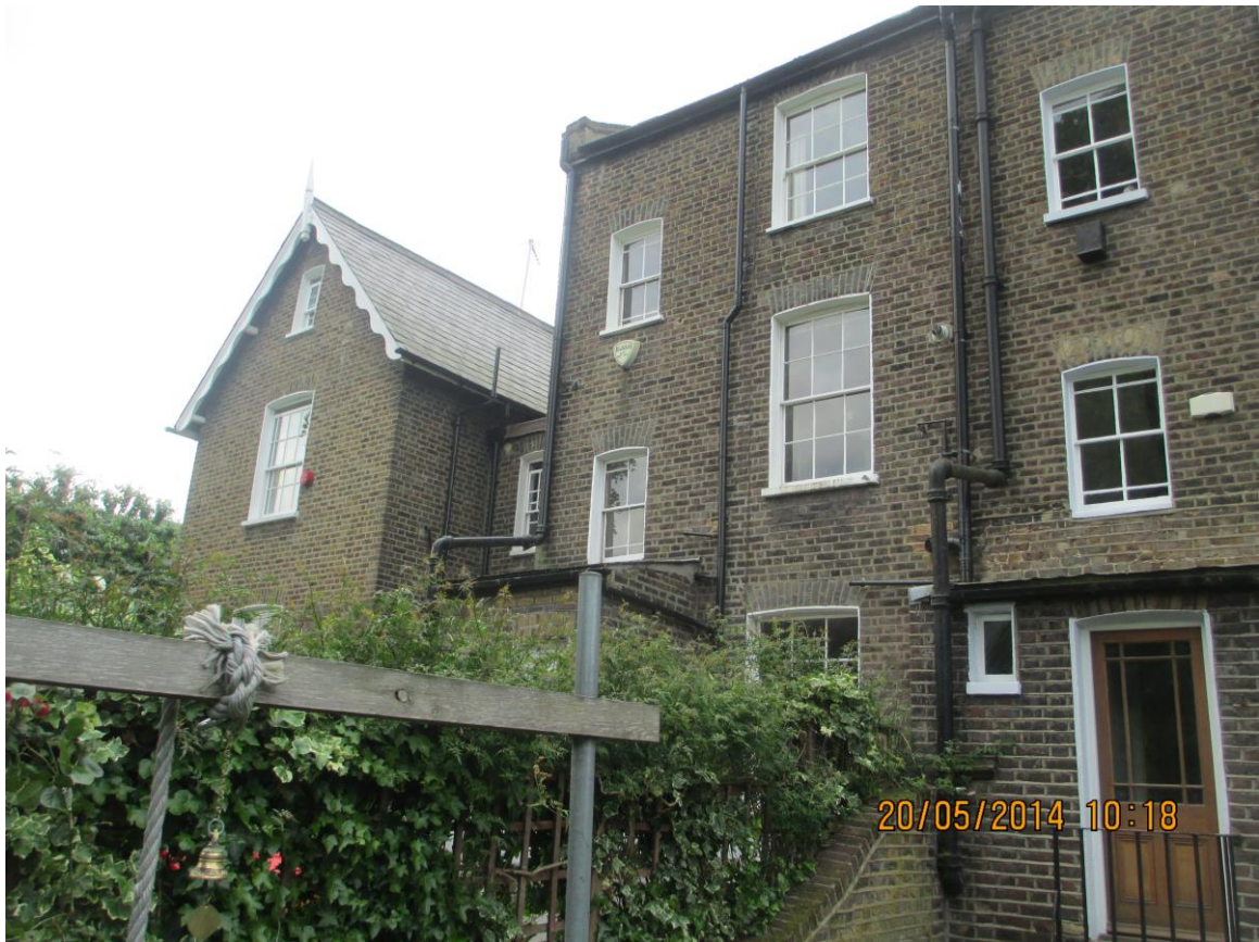
Image 4 – View of rear elevation of the adjoining property at no. 6 St Paul's Road
