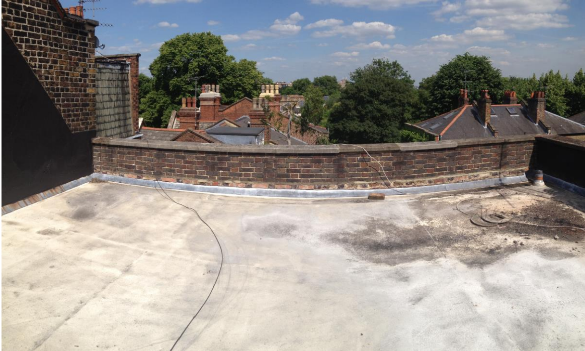
Image 3: View from existing roof
