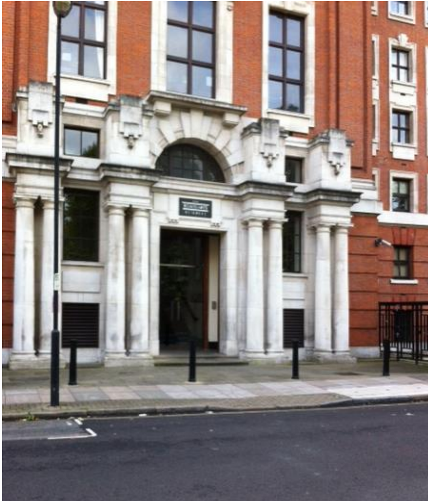
Photo 2: Main entrance Beaux-Arts Building
