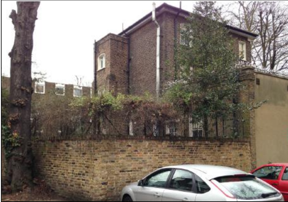
Image 2: Rear elevation from adjoining residential parking
